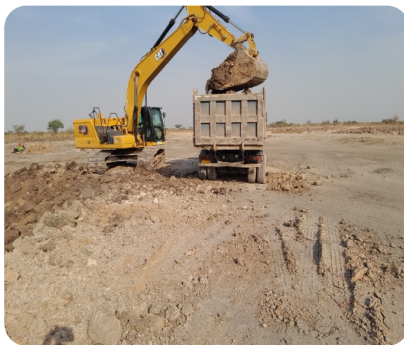
Dugout expansion work underway to secure a reliable, year-round water source for a Saha partner community.
